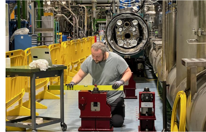
HL-LHC magnet support alignment
